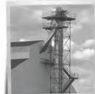
BUCKET ELEVATOR LEGS
