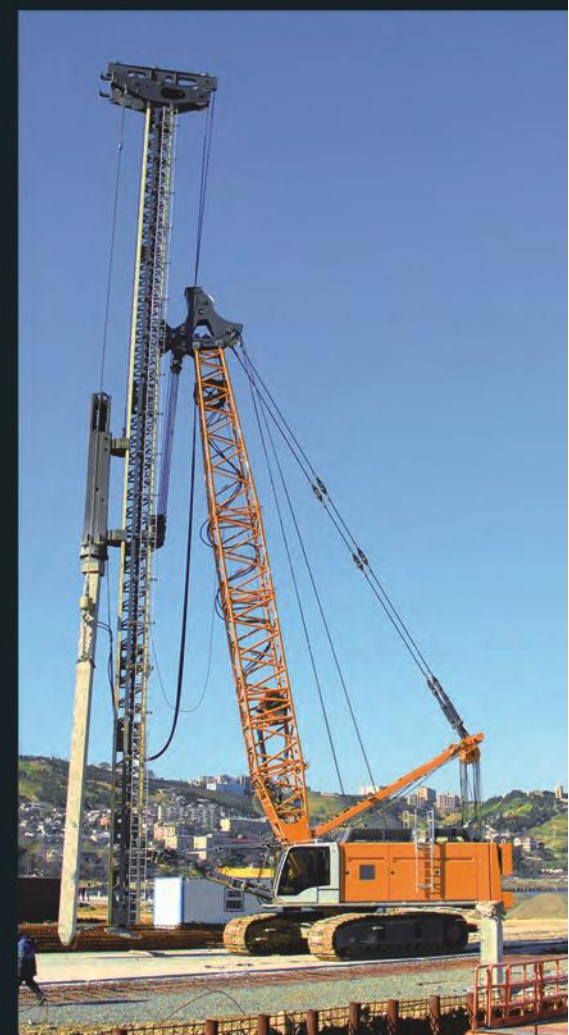
The Liebherr LRB 255 on site and in operation in Quebec, Canada
