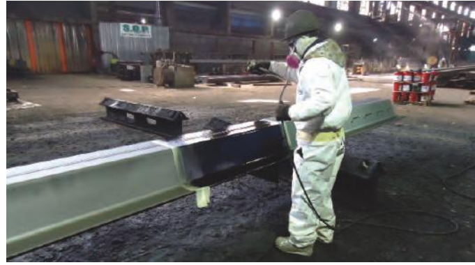
Application of corrosion coating to existing structurally fabricated steel.
