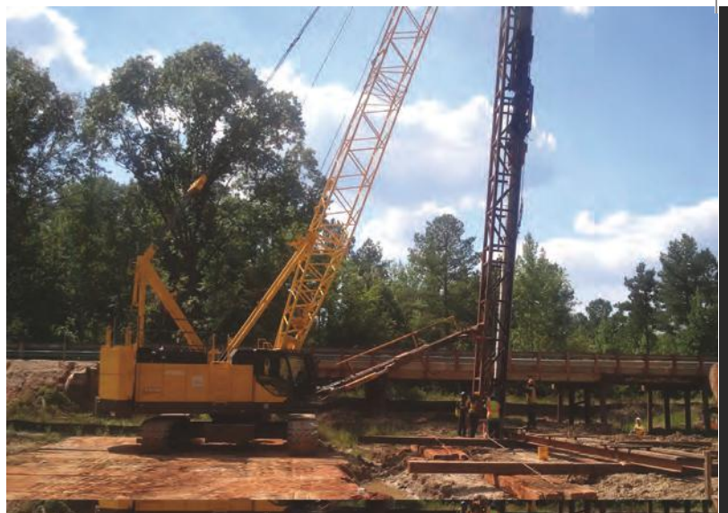
Driving 16-inch test pile in Attala County on Hwy 12. There were 10 different bridge sites on this project
