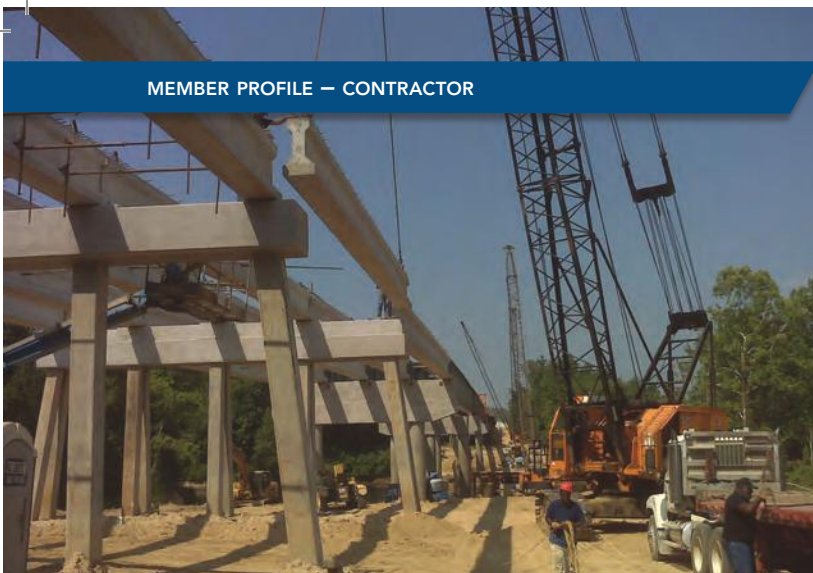
Hanging beams in Marion, Co. for a bridge over the Pearl River on Hwy 43
