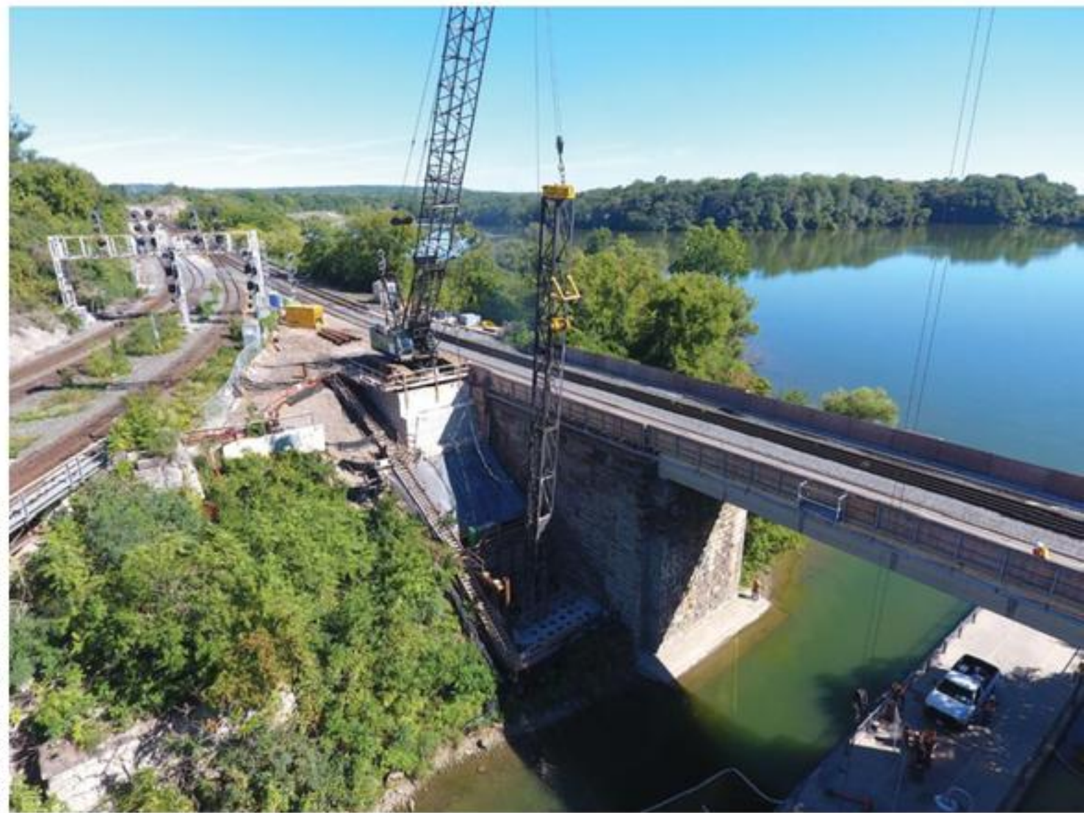
BERMINGHAM FOUNDATION SOLUTIONS
